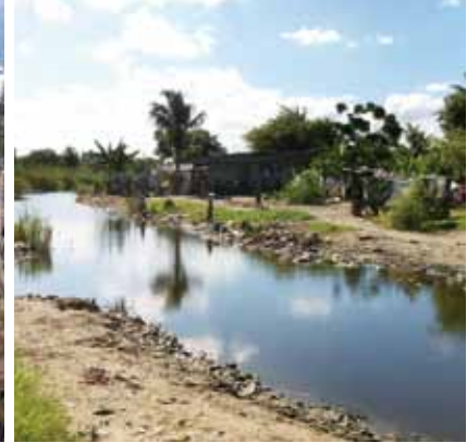
Drainage Rehabilitation Works Beira, Mozambique
