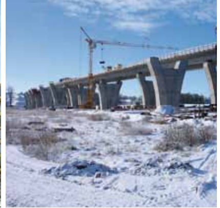
Construction of motorway A14, Germany
